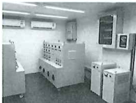
Refrigerator - Energy Room
